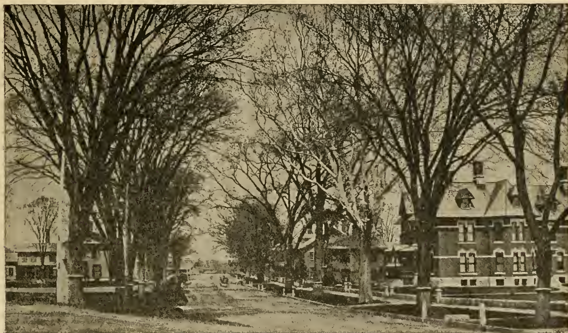
MAIN STREET, CONCORD, AT THE NORTH END.
